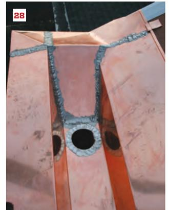
met the trough, we bent a ½-inch leg that would form the soldered connection. To install these pieces, we slipped the legs under the liner trough, molded the upper portion to the roof, the crown-molding cap, and the gutter return, and soldered the seams (28).
