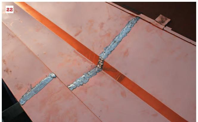
the drip edge and settled the panel into the trough (21), then secured it on the roof side with 1 ½-inch-wide copper cleats 24 inches on-center, fastened to the sheathing with 1 ½-inch-long copper nails. We overlapped the next liner panel by 3 inches, then soldered the seam (22) (see Soldering Seams, facing page). With two panels in place at one end, we switched sides and installed two panels at the other end.
