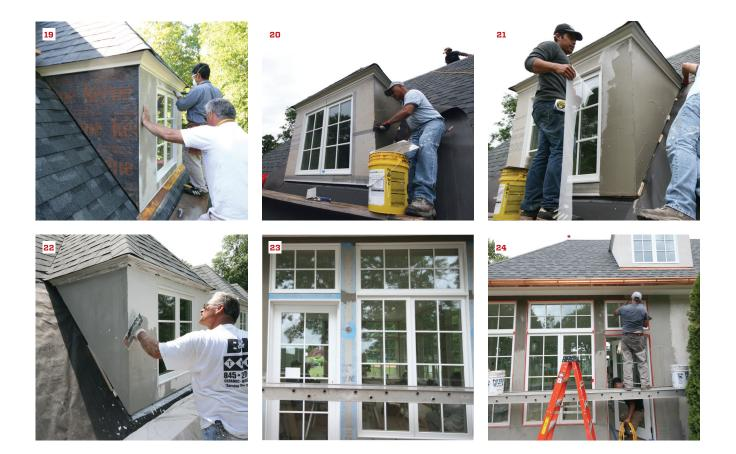
the window frame, then ran a strip at the head flashing. After finishing each window, we rolled all of the tape with a J-roller to set the adhesive.
