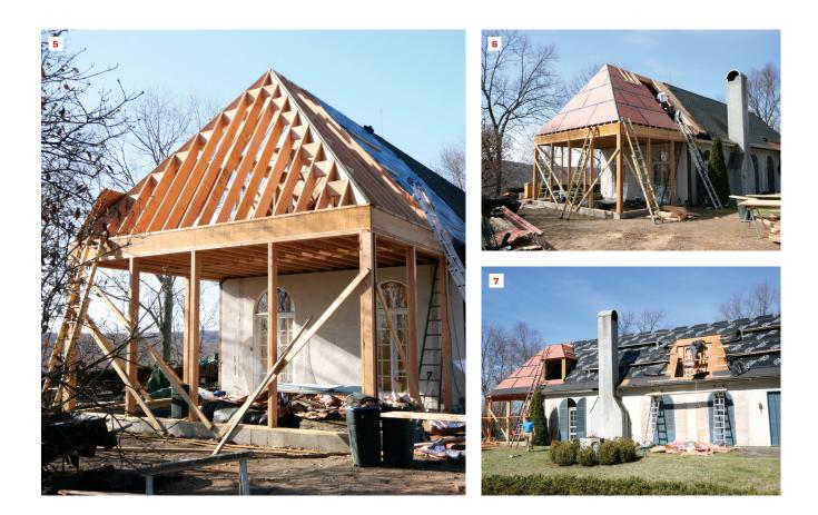
used LVL for end joists and doubled it up to serve as a header on the long wall of the sunroom. For bridging at midspan, we used solid 2x12 blocks.
